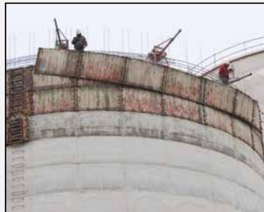
Workers from McPherson Concrete move the form on the new 348,000-bushel bin in Tampa.
